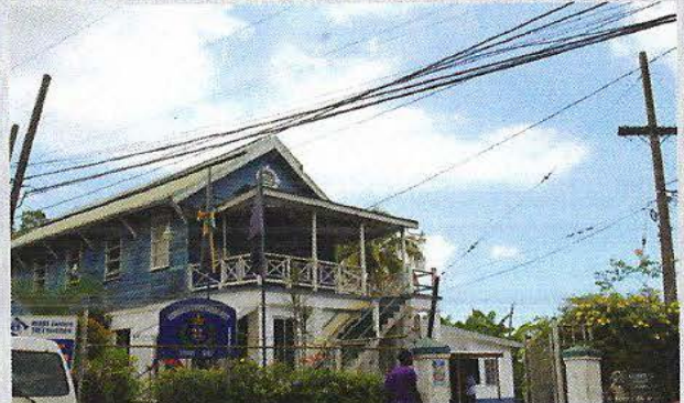
Police Station in Stony Hill and Courthouse to be refurbished.
