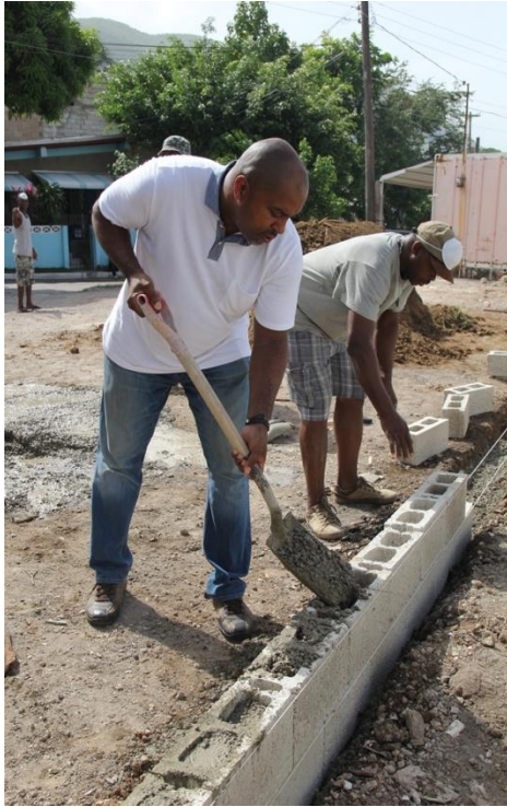
Pouring cement in a wall being constructed for a floral park in Nannyville
