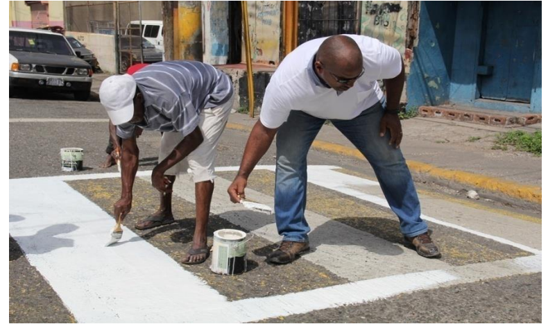
Painting a pedestrian crossing on Slipe Road in Cross Roads
